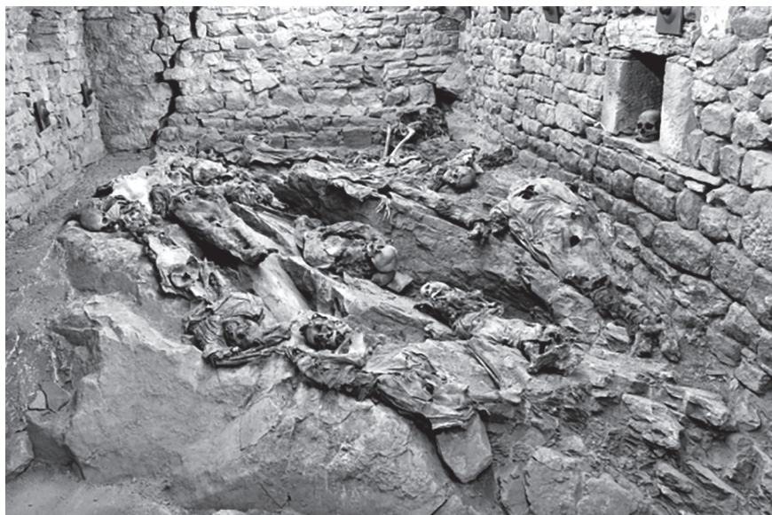
Fig. 1. Loopholes in the wall of the crypt allowing a proper ventilation of the burial site.
