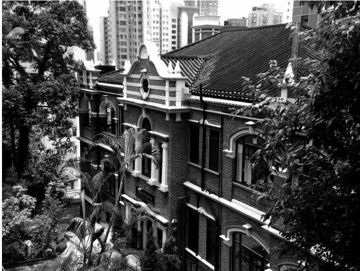
Fig. 1- The Hong Kong Museum of Medical Sciences, housed in a well-preserved 100 year-old Edwardian Style building, a protected monument. Its architecture is in sharp contrast to the many typical high rises which now surround it.
