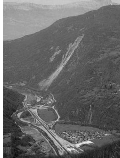
Figure 20 - Zone of impact of Séchilienne rockfall
