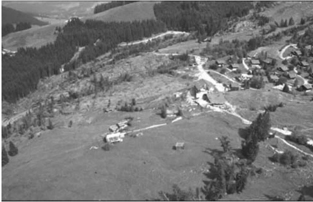
Figure 13 -Lower part of Chlöwena landslide and destroyed Falli Hölli village. The lower part of the slide evolved in a mudslide to form a dam in the nearby river
