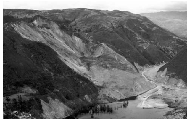
Figure 18 - View of La Josefina landslide dam, some months after breaching. A deeper artificial channel is excavated to decrease the level of the residual lake
