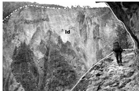
Figure 7 - SE-NW view towards Dukur Pokhari rockslide (ld, dashed-dotted line); position: 1.5 km west of Bhratang, alt. 2900 m; photograph: J. T. Weidinger 1993
