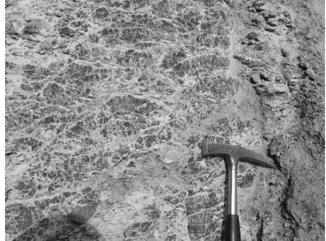
Figure 2 - Crushed jigsaw facies of the rock slide material. The components have perfect fitting, but are completely loose and can be dugged out by hand
