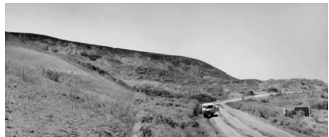
Figure 8 - Ak-Shaluu landslide – view to main scarp and displaced material with new dirt road – picture taken in July 1999 (for position and look direction see Figure 7)
