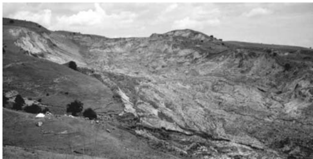
Figure 4 - Landslide Kotchkor-Ata – view to main scarp (width ca. 500m) – picture taken in July 1999
