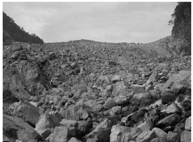
Figure 6 - View over the carapace of the Tsatichhu rock-avalanche deposit to the dam crest (the deposit was around 110 m deep) with seepage evident. The carapace and upper interior properties contrast are interpreted to have played a key role in the dam failure
