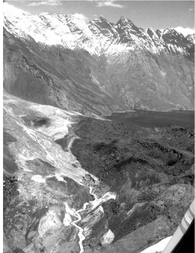
Figure 2 - Helicopter view on the proximal (northern) part of the Usoy Dam
