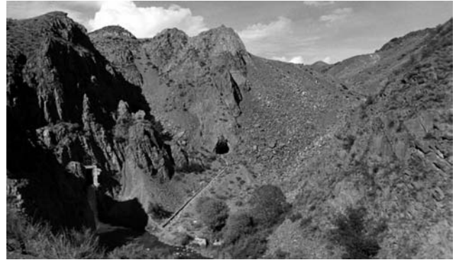
Figure 4 - The Burlykia experimental blast-fill dam. Adit at the base of the right slope was made to investigate seismic effect of the explosion on the underground structures
