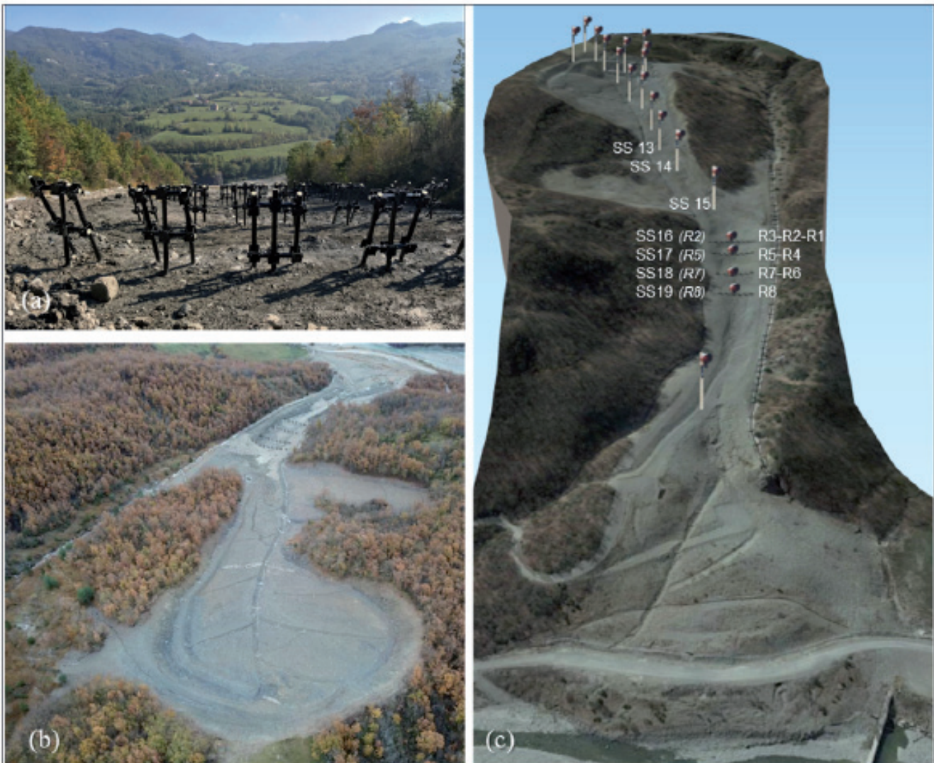
Fig. 6 – Field and aerial views of ground reshaping and MTS finalization as integral part of all other slope consolidation intervention. LEGEND: (a) Upslope to downslope field view. (b) Upslope to downslope aerial view. (c) Downslope to upslope aerial view with labels and relative position of monitored tripods (R1 to R8) and topographic monitoring prisms (SN13 to SN19)
