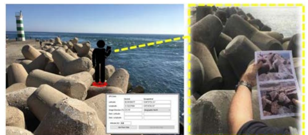
Fig. 1 - Visual observation technique used in each breakwater.
