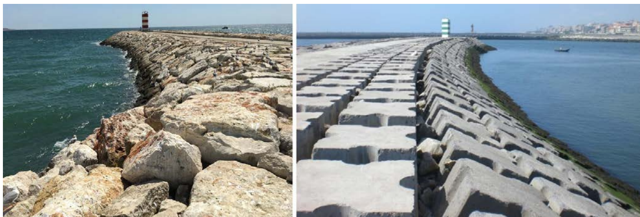
Fig. 1 - Typical rubble-mound breakwaters with armour layers composed of: Left: rock units; Right: artificial units.
