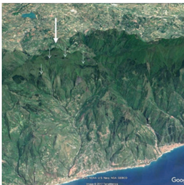
Fig. 11 - View of Caloria M.t (arrow); in the northern slope there are numerous dolina shaped depressions, concentrated due to piping phenomena (thin arrows), at the rotational and lateral spreads and sliding bands. Coordinates: 39°31'21.04"N15°55'38.41"E; 39°42'10.85"N16°10'12.90"E; 39°30'18.52"N16°17'16.12"E; 39°27'12.48"N15°59'05.48"E
