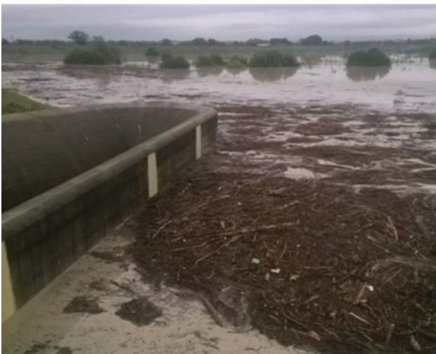
Fig. 7 - Aerial view of the dam (top), accumulation of the driftwood at the right duckbill spillway and condition of the reservoir at 18:13 of October 13 th 2014 (bottom)
