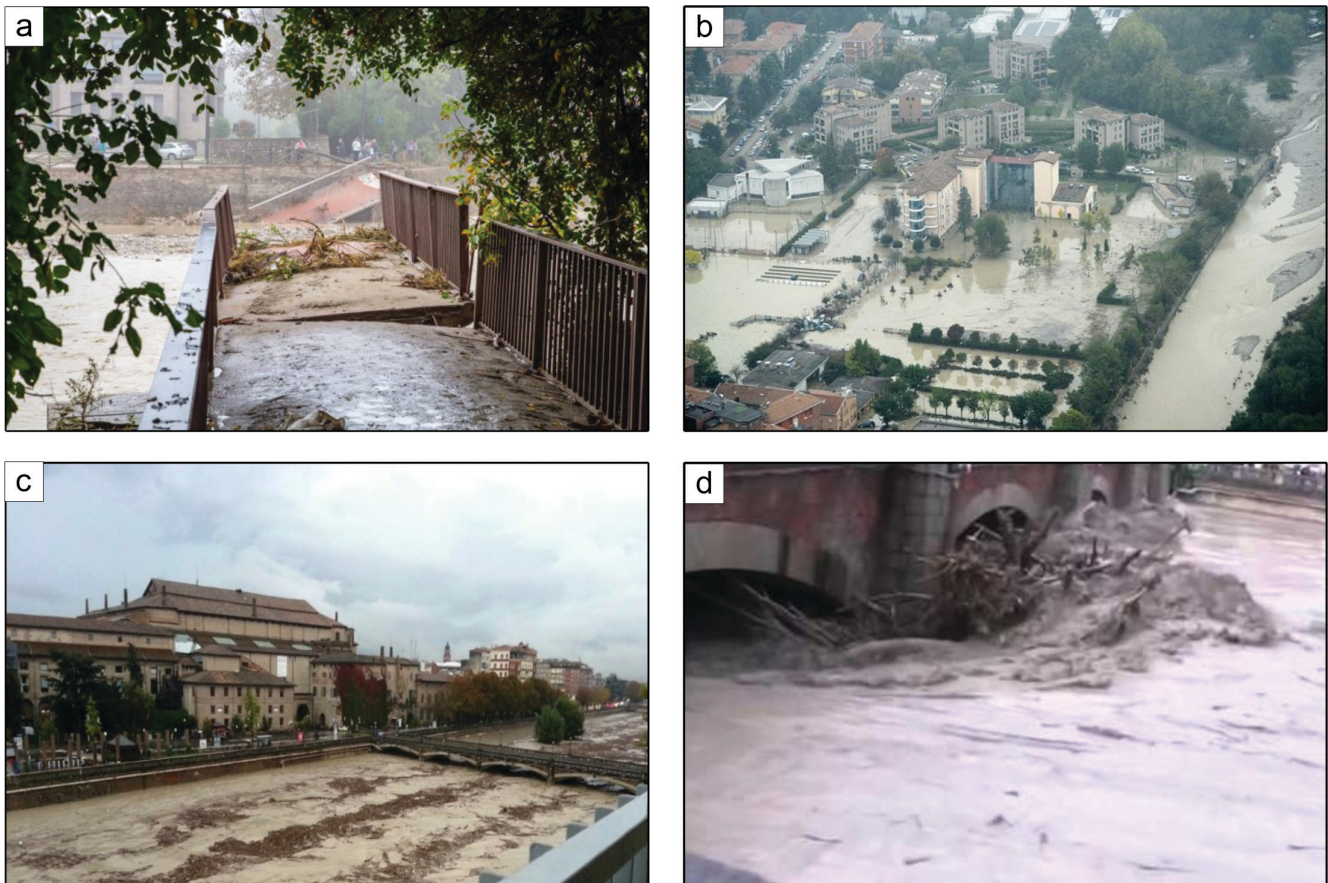
Fig. 4 - October 13 th 2014 flood event: a) initial phases of the historical pedestrian bridge collapse; b) residential neighborhoods flooded by the Baganza river; c) urban reach of the river Parma downstream of the confluence with the Baganza river; d) bridge piers with wood debris
