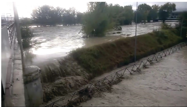
Fig. 5 - Incipient breaching in the river Parma levee
