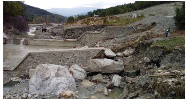
Fig. 16 - The Sassi Neri check dam after the flood event (from downstream). The flow circumvented and damaged the structure on the left
