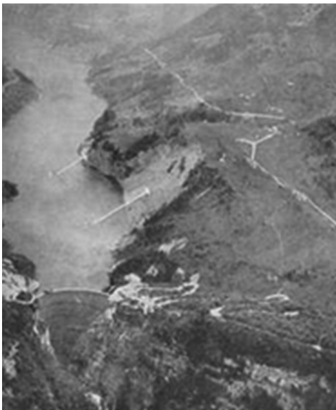
Fig. 15 The 4 th November 1960 landslide on the left reservoir slope
