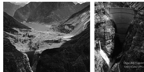
Fig. 6 - The dam reservoir after the landslide
