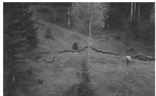
Fig. 14 - Part of the perimetral M-shaped fissure opened on October 1960
