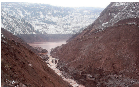
Fig. 8 Eroded breach in the debris deposit of the Hattian Bala landslide below the artificial spillway. Note the landslide scars in the background and the former level of Karli Lake marked by the snow line. Photo taken on February 10, 2010 by Dr. Kausar from the Geological Survey of Pakistan
