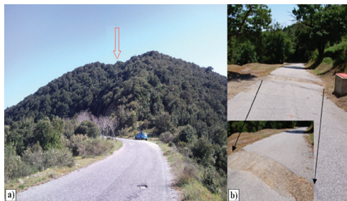
Fig. 3 - a) Top of the Mt. Granieri slope. The arrow points to the double crest, visible in the upper part of the relief, where the future landslide scarp will be located; b) Rupture surface (and related detail) along the internal Caulonia-Nardo di Pace provincial road. On the right-hand side, the monitoring station whose location is shown in Fig. 2
