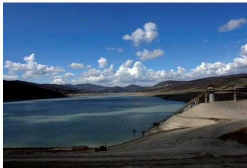
Fig. 1 - General view of Sioni earth dam upstream wall
