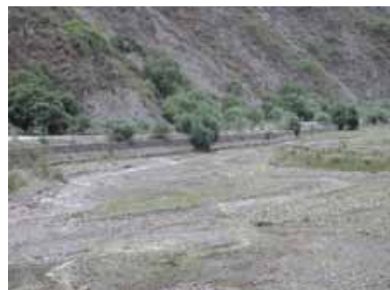
Fig. 8 - The longitudinal defence work built on the left bank of Río Toro, downstream the confluence with Río Candado. It needs frequently to be raised, due to the aggradation of the riverbed
