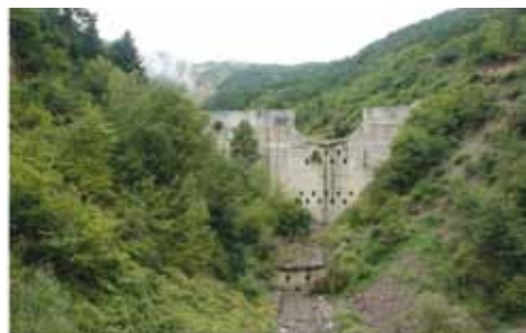
Fig. 4 - Check dam for prevention debris flow in Heishui, Sichuan
