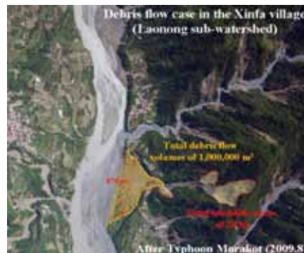
Fig. 15 - The debris flow hazard in Xinfa village in the Laonong river watershed in Gaoping watershed after Typhoon Morakot
