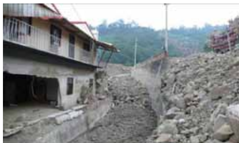
Fig. 18 - Building was damaged by debris flow (photo: Meei-Ling Lin)
