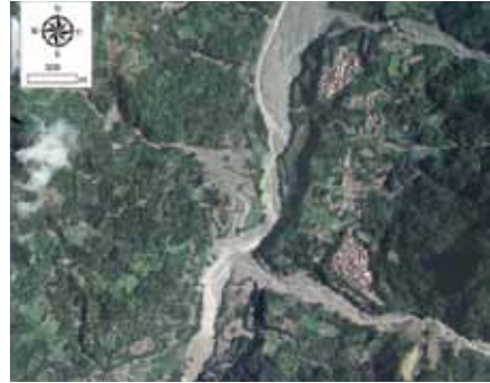
Fig. 9 - Aerial photo of Dakanuwa village after typhoon Morakot (provided by NCDR)
