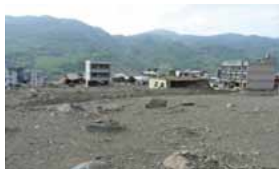
Fig. 6 - Debris covered entire Nanshalu village (photo: Meei-Ling Lin)
