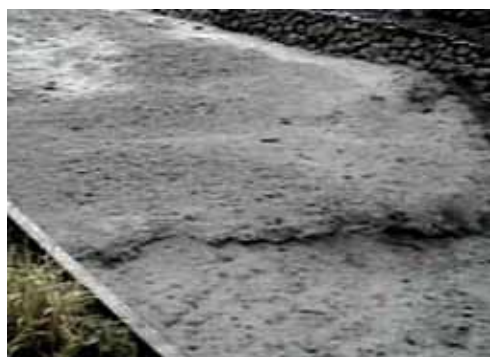
Fig. 5 - Debris flow image in Aiyuzih creek, Shenmu station
