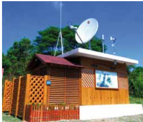
Fig. 2 - Instrumental cabin of Jiufen-ershan station in Nantou County.
