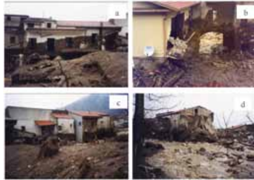
Fig. 6 - Typical examples of damage caused by the Ioffredo debris flow
