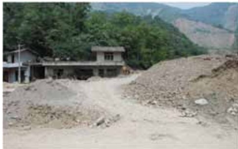
Fig. 3 - Houses destroyed by the September 24, 2008 debris flow
