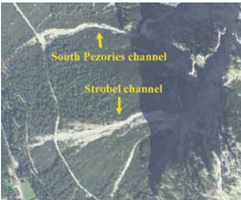
Fig. 2 - Overview of the two debris flow channels at Fiammes
