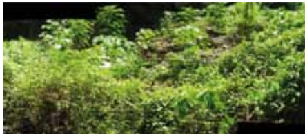
Pic. 2 - Ground with serious erosion on left bank hill
