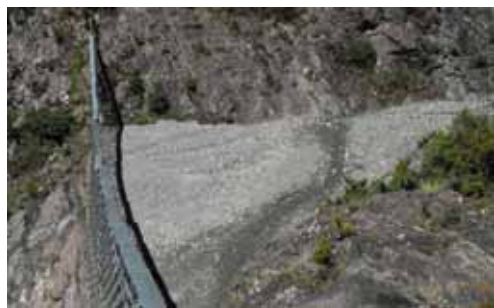
Fig. 9 - Lateral view of the barrier filled in Erill
