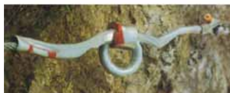
Fig.10 - Energy absorption of the single brake rings
