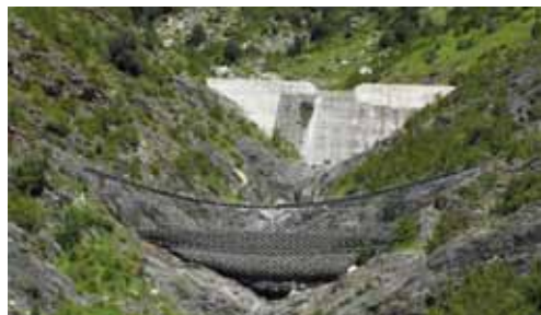
Fig. 8 - Frontal view of the barrier filled in Erill
