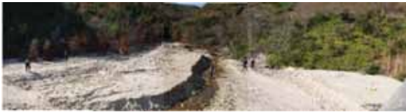
Fig. 17 - Sediment deposition caused by the upstream check dam on the Hachimandani River (View from downstream to upstream direction on December 8, 2009)
