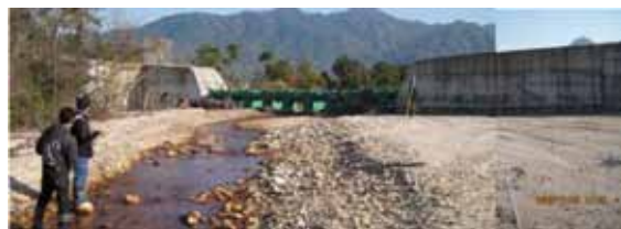
Fig. 23 - Sediment deposition caused by the downstream check dam on the Hachimandani River (View from upstream to downstream direction on November 25, 2009)
