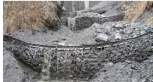
Fig. 12 - Filled multi-level barriers in the Merdenson torrent, Switzerland
