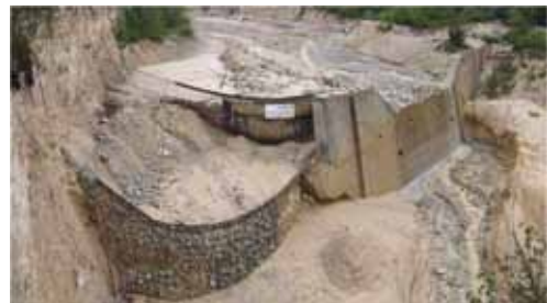
Fig. 13 - Net barriers as a repair and deviation construction in the Illgraben, Switzerland
