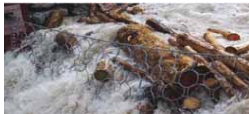
Fig. 16 - Net barrier against driftwood
