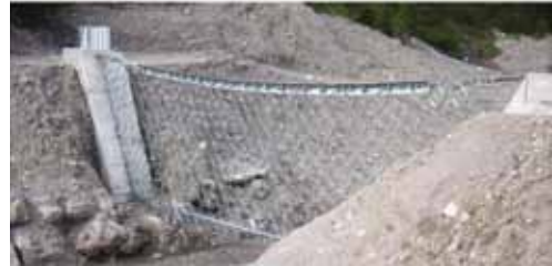
Fig. 11 - Debris flow barrier at the Schlucher Ruefe torrent, Liechtenstein
