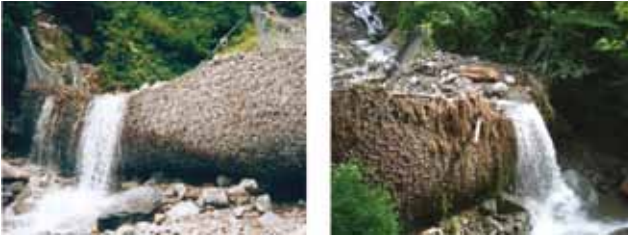
Fig. 1 - Debris flow barriers 1998 in Aobandani, Japan (left, 750 m 3 retained, deflection 2 - 3 m, remaining barrier height reduced from original 5 m down to 3.5 m) and 2008 in Villar Sautoreglia, Italy (right, 1500 m 3 retained). Post-event material (water and sediments) goes over the barriers
