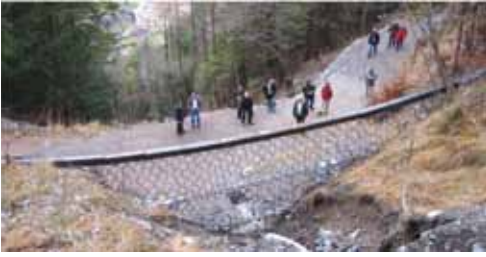
Fig. 9 - Debris flow barrier in the Engler torrent, Berner Oberland, Switzerland
