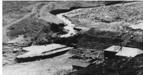
Fig. 6 - The dam opening after the 1973 debris flow in the Mynzhilki tract
