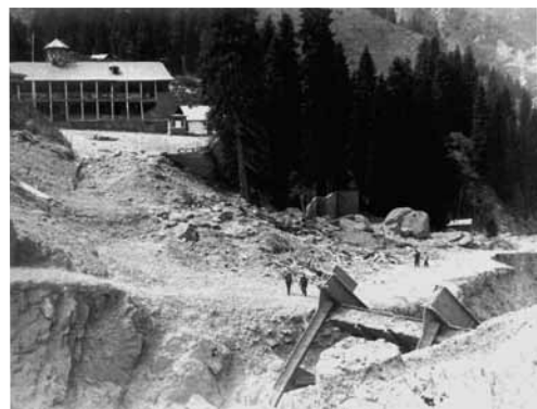
Fig. 7 - The open-type dam destroyed by the 1973 debris flow
