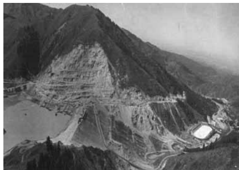
Fig. 8 - The debris-flow reservoir filled by the 1973 debris-flow mass in the Medeo tract
