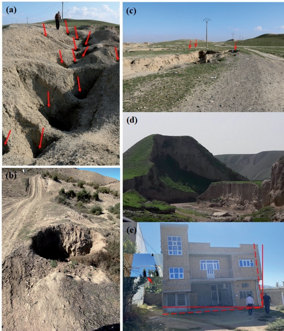
Fig. 1 - a) Abundance of loess caves on Kalaleh-Maraveh Tappeh road b) A loess cave developed near the Cheshmehli village road c) Loess caves along the power transmission line around Maraveh Tappeh d) Typical landslide developed on the loess plateau in Golestan Province e) Differential settlement of residential building in Feraghi city, and Bending of gas supply pipe of houses in Feraghi city due to loess collapse
