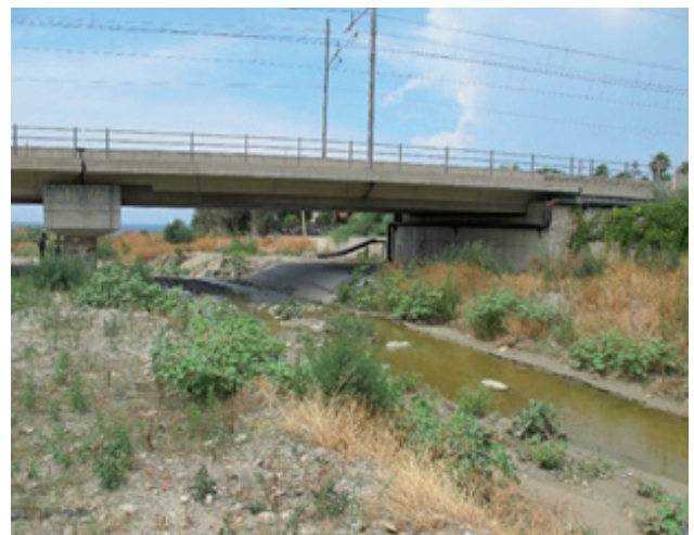
Fig. 11 - Concrete slab near the railway bridge pile
