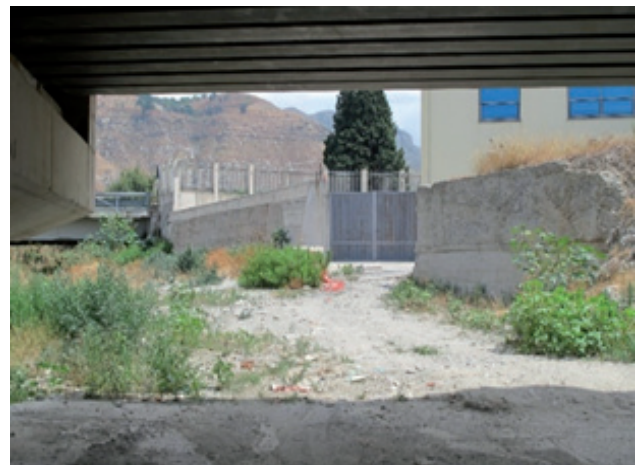
Fig. 10 - Levees openings downstream of the highway bridge near anthropized areas.
