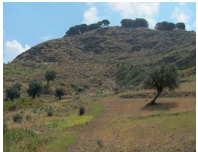
Fig. 6 - Active landslides near the Scillupia reservoir
