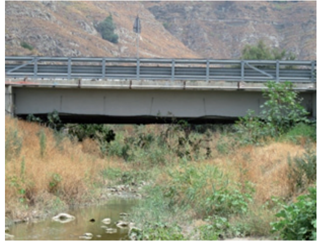
Fig. 9 - Partial obstruction of the river section below the highway bridge due to vegetation and aggradation
