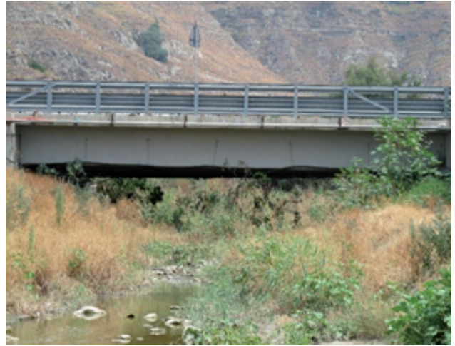
Fig. 9 - Partial obstruction of the river section below the highway bridge due to vegetation and aggradation
