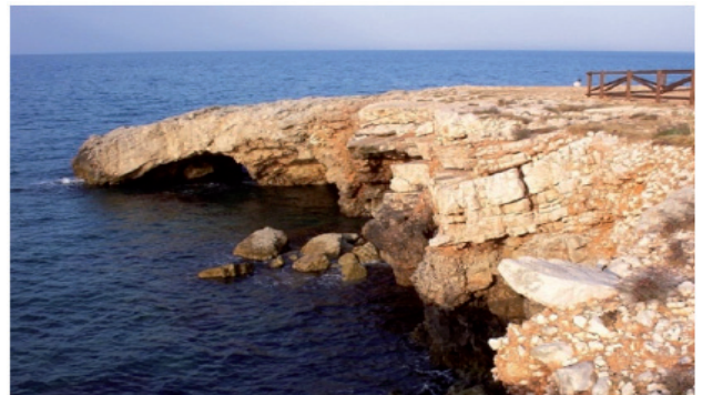
Fig. 7 - Planar failures along bedding planes in the proximity of "Grotta Chiar di luna" cave (northern coastal stretch of Polignano a Mare)
