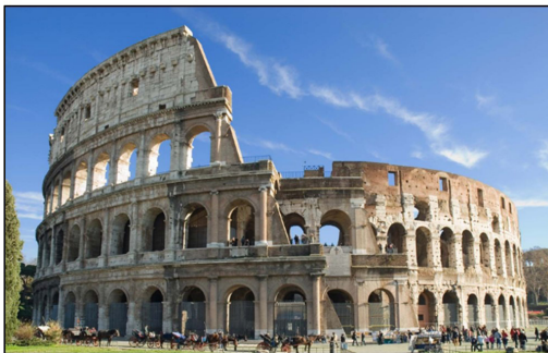
Fig. 4 - The building foundations of Ancient Greeks and Romans: foundations of the Temple of Juno in Agrigento, Italy (top) and the Coliseum, Rome (bottom)
