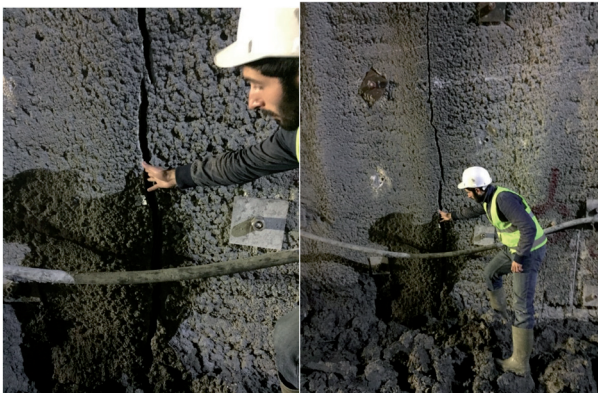
Fig. 11 - Cracks in shotcrete and failures in bolts
