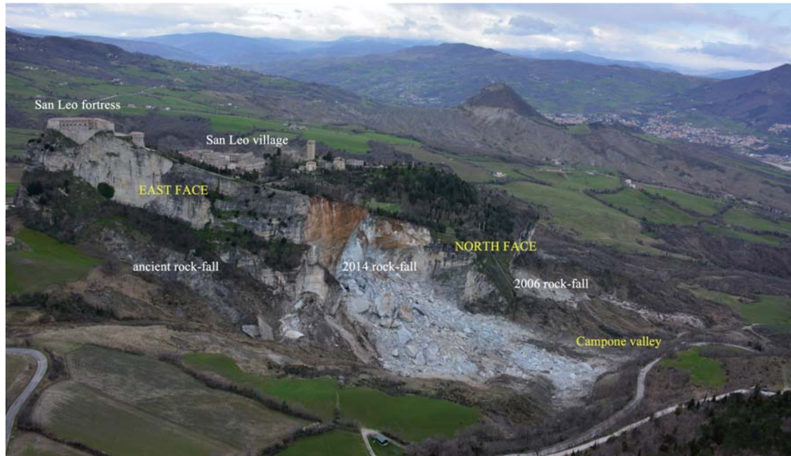
Fig. 4 - Panoramic photo from helicopter after the 2014 event at the north-east edge of the cliff. The landslide generated an extensive and thick rock avalanche deposit invading the Campone valley. On the right, along the north side of the cliff, we can appreciate the 2006 rock-fall deposit at the foot of the wall. Finally, an ancient huge landslide rests at the foot of the east face
