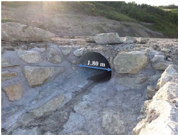
Fig. 13 - The steel pipeline for bypassing the 2014 landslide deposit
