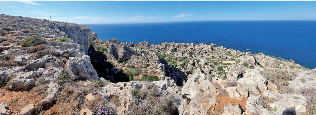
Fig. 9 - Panoramic views of the cliff at Sopa promontory in the Island of Gozo which is involved in a lateral spreading responsible for the dislodgment of huge blocks of UCL over the BC formation causing their back tilting and toppling all along the coastal slope
