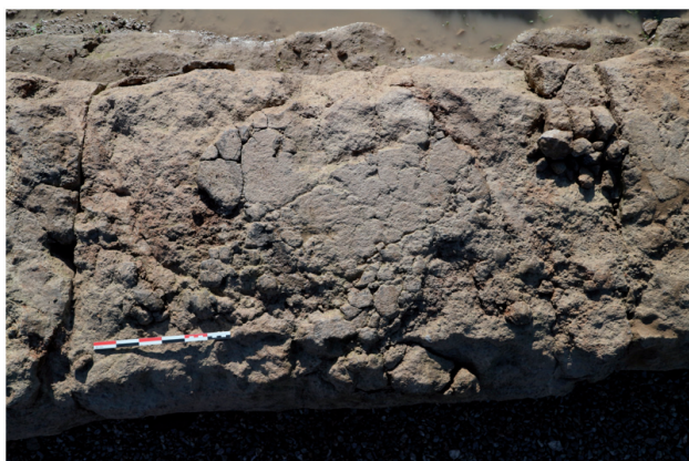
Fig. 12 - Phenomenon of erosion of soft limestone due to the effect of frost (DAI-Athen archive)
