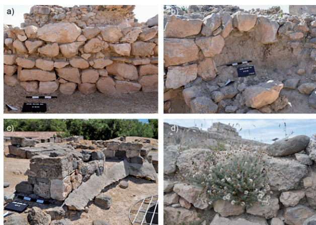
Fig. 9 - Types of damage a) Washed-out joints. b) Undermined foundation and fallen stone. c) Detached cement mortar. d) Vegetation
