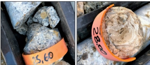
Fig. 4 - Details of the material extracted from the core drilling performed
