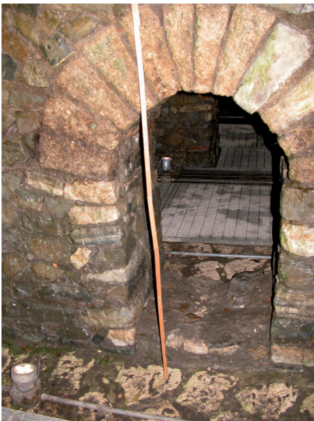
Fig. 10 - The opening in tunnel n. 1 consists of ashlars of travertine
