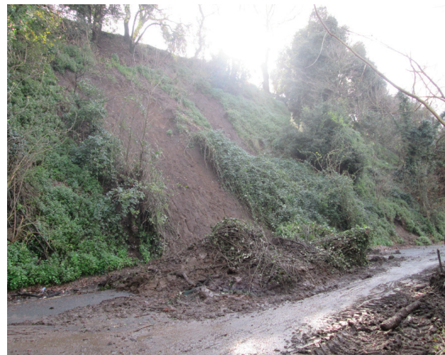
Fig. 11 - Examples of landslides triggered in Rome by the exceptional rainfall event of 31 Jan.-2 Feb. 2014: translational slide along Via della Marcigliana
