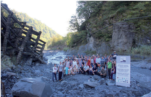
Fig. 6 - The destroyed structure in the Duruji River upstream the Kvareli town (Photo by I. Kargapolova)
