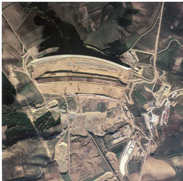
Fig. 8 - Aerial view of the Locone dam during construction (1970s)
