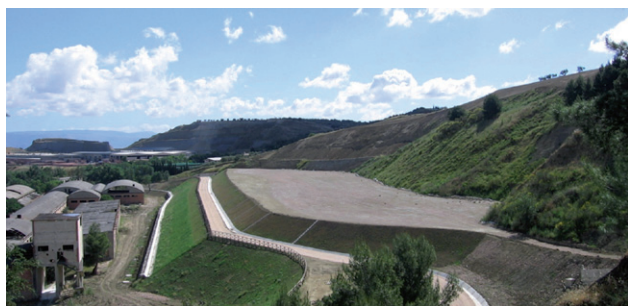
Fig. 9 - Landslide remediation works in Lucera (1980s)
