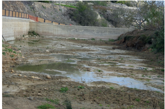
Fig. 2 – The inner reservoir at Chadwick Lakes in early November, 2020.
