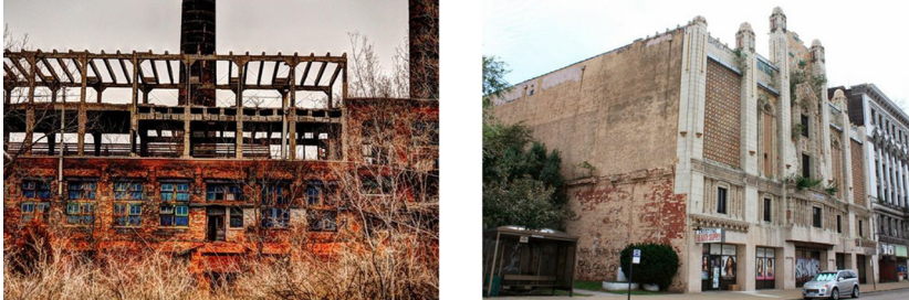
Fig.1: on the left, an abandoned meatpacking plant; on the right, the recently demolished Majestic Theater in East St. Louis (source: St. Louis Newspaper).
