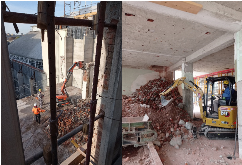
Fig. 3 Workers and machinery operating on a demolition site. Source: photos by the author.
