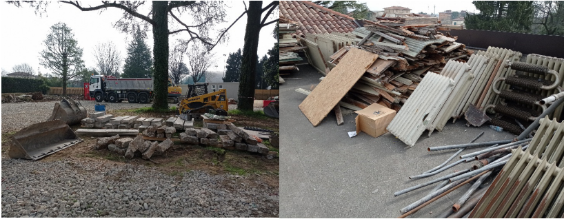
Fig. 2 Piles of materials being sorted on site for reuse or disposal. Source: photos by the author.
