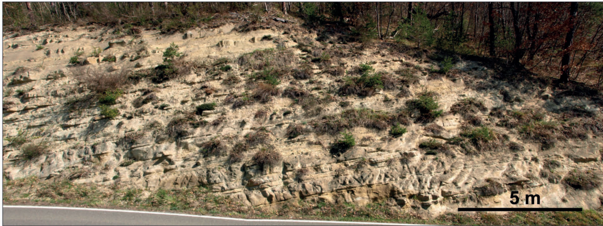
Fig. 19 - Detail of the thick- to very thick-bedded, amalgamated sandstones beds of the Cassinasco Fm cropping out along the road Torre Bormida-Cravanzana.
